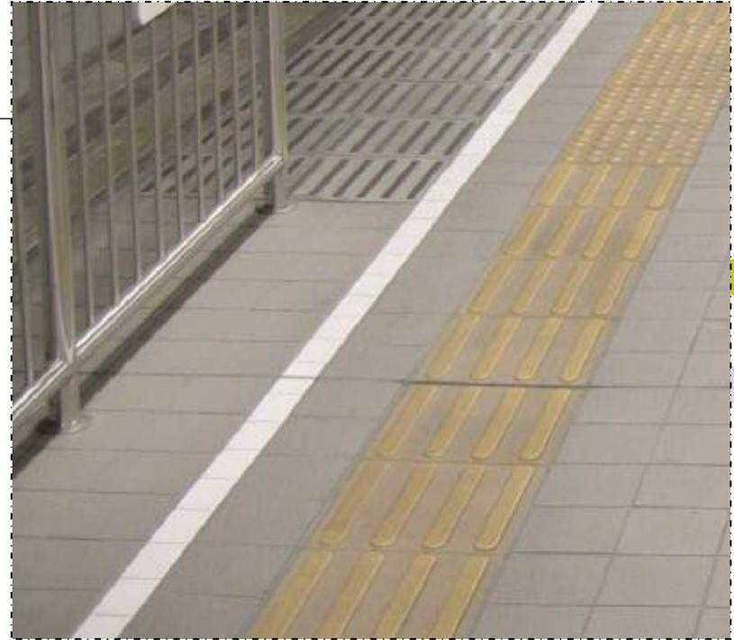
Smooth/continuous/clean/neatly warning Braille guide block and kerbed cut
