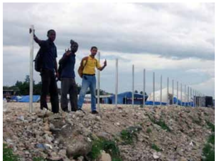
Start of building a security fence around the tent site
